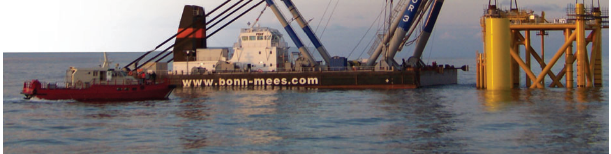
Matador 3 in action on open-water construction site
